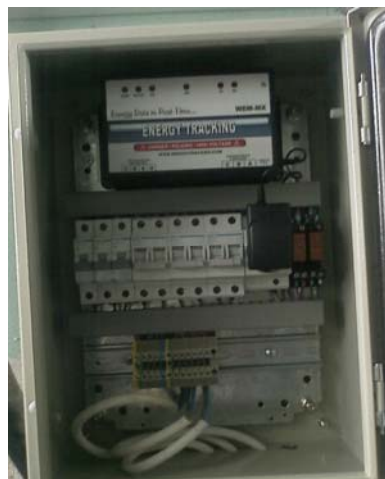
Fig. 1 – WEM-MX AMR installation to Greek School
